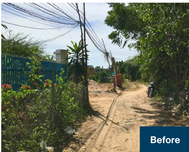
Figure #: To provide consistently safe and reliable power access to the local community, TBC has replaced the temporary wooden power poles of transmission lines with concrete ones in certain remote areas.
